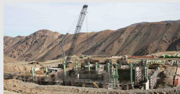
Los Bronces Expansion – SAG and Ball Mill Foundations
