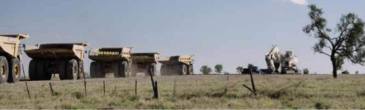
Left: Preparing to excavate the Dawson pit.
